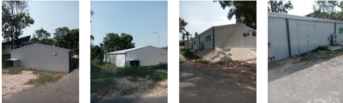
Figure 1. BSF House (pilot) in RIBE
